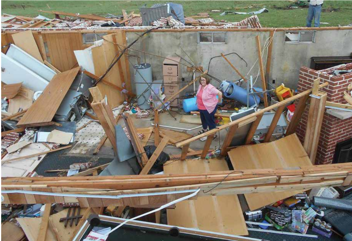
Deb Wood surveys the damage after an EF4 tornado destroyed her home May 25, 2016. She had sought shelter in the basement. With her was a “grab-and-go” box of financial records.
