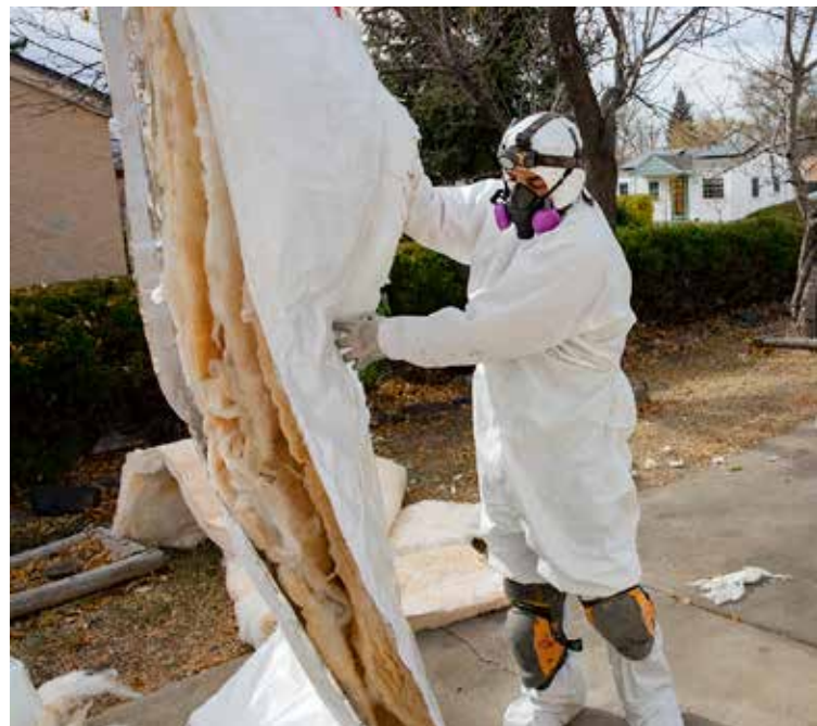
A worker handles insulation during an Energy Resource Solutions project.
